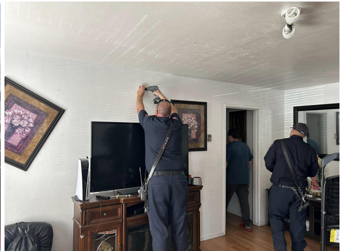
HFD Firefighters install smoke detectors
